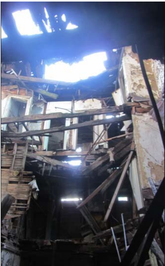
Figure 23. 28 West 130 th Street Interior Roof Collapse. October 2012. Photograph by author.
